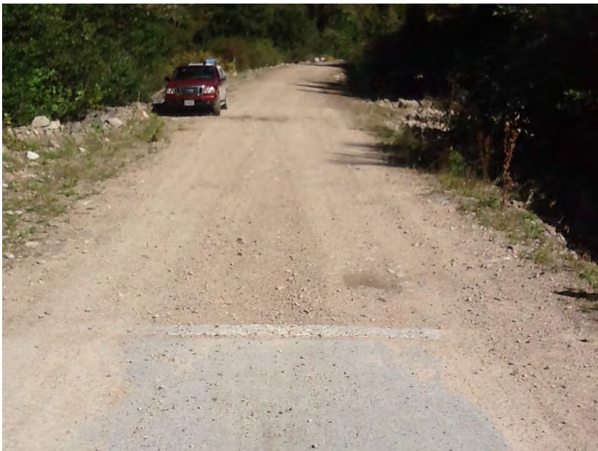
Left approach facing away from structure
