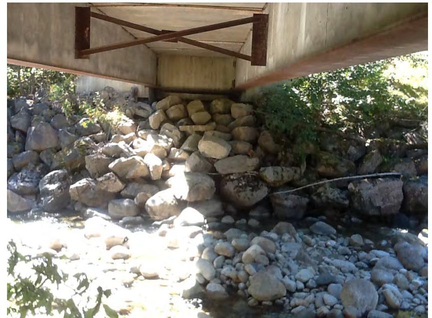
Right Bank Abutment when facing downstream
