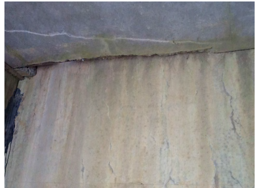
Right Bank Abutment when facing downstream
