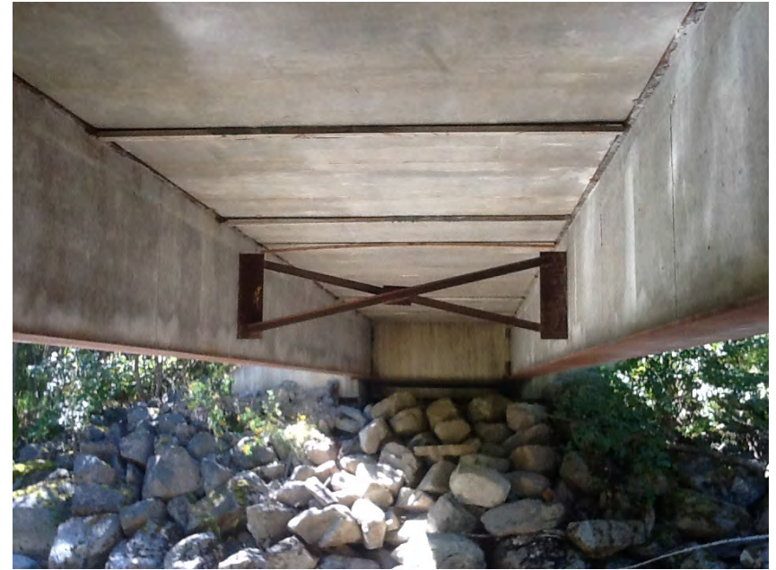
Underside of bridge
