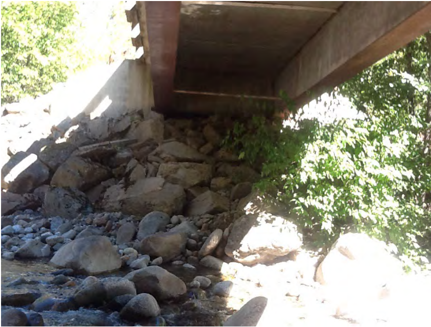
Left Bank Abutment when facing downstream
