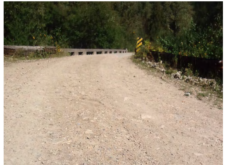
Right approach facing structure
